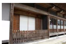
293_外観正面玄関001
