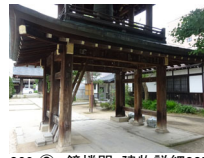
029_③ 鐘樓門・建物詳細007
