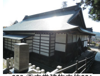
003_②本堂建物本体001
