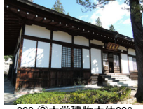
008_②本堂建物本体006
