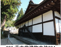
006_②本堂建物本体004
