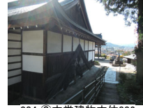
004_②本堂建物本体002
